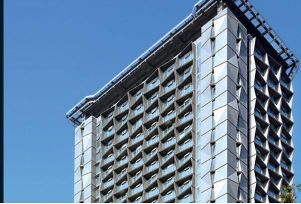
**ALPOLIC™ A2 aluminium composite panels consist of two 0.5mm thick aluminium cover sheets which are applied to a non-combustible (UK: limited-combustible) mineral core in a fusing process. They can be supplied up to a width of 2m, which is unique worldwide.**
