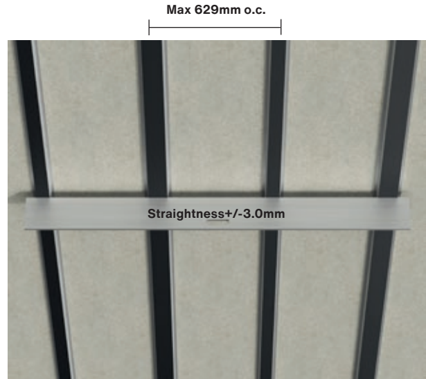
Straightness of substructure
